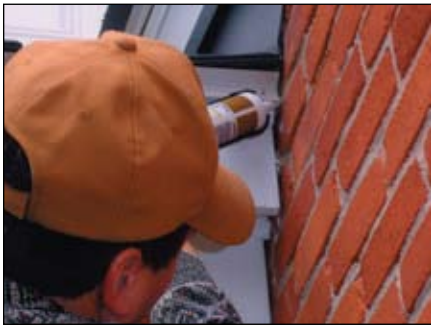
Dreisacker applies caulk to seal possible bat entry points.
