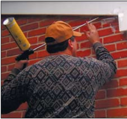
Dreisacker often uses a sealant foam to close openings in structures.
